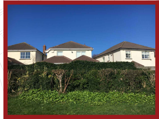
EXISTING WALL RETAINED. TYPICALLY 1.8M HIGH BREEZEBLOCK WALL AND BRICK WALL
