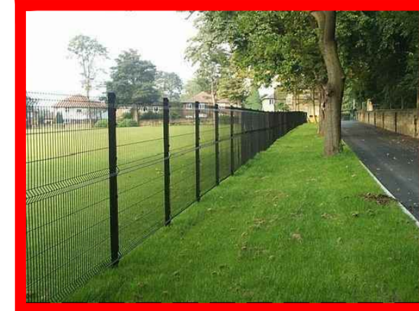
MIN. 1.8M HIGH WELDED MESH PANEL FENCE
